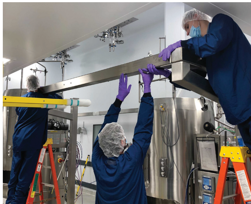
Ernest D. Menold, Inc. employees installing an exhaust system on roof.
