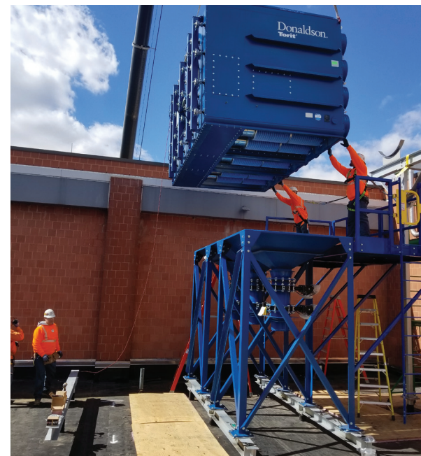
Ernest D. Menold, Inc. employees installing an exhaust system on roof.
