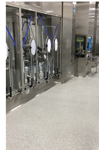
Installed skirting trim around base of equipment
