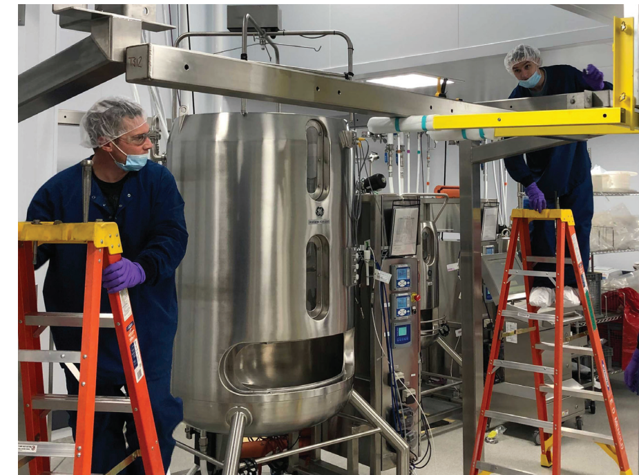
Ernest D. Menold, Inc. installing a platform around bioreactors in 2021.
